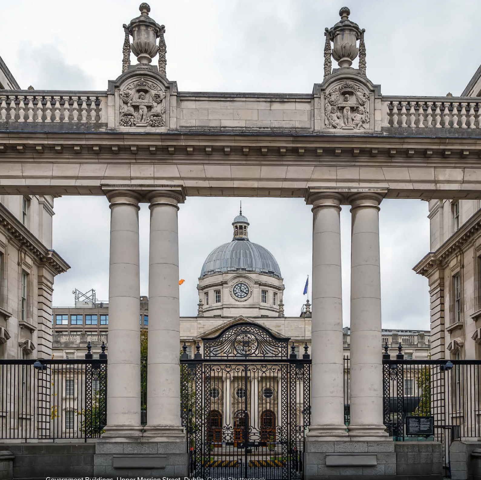
Government Buildings, Upper Merrion Street, Dublin. Credit: Shutterstock
